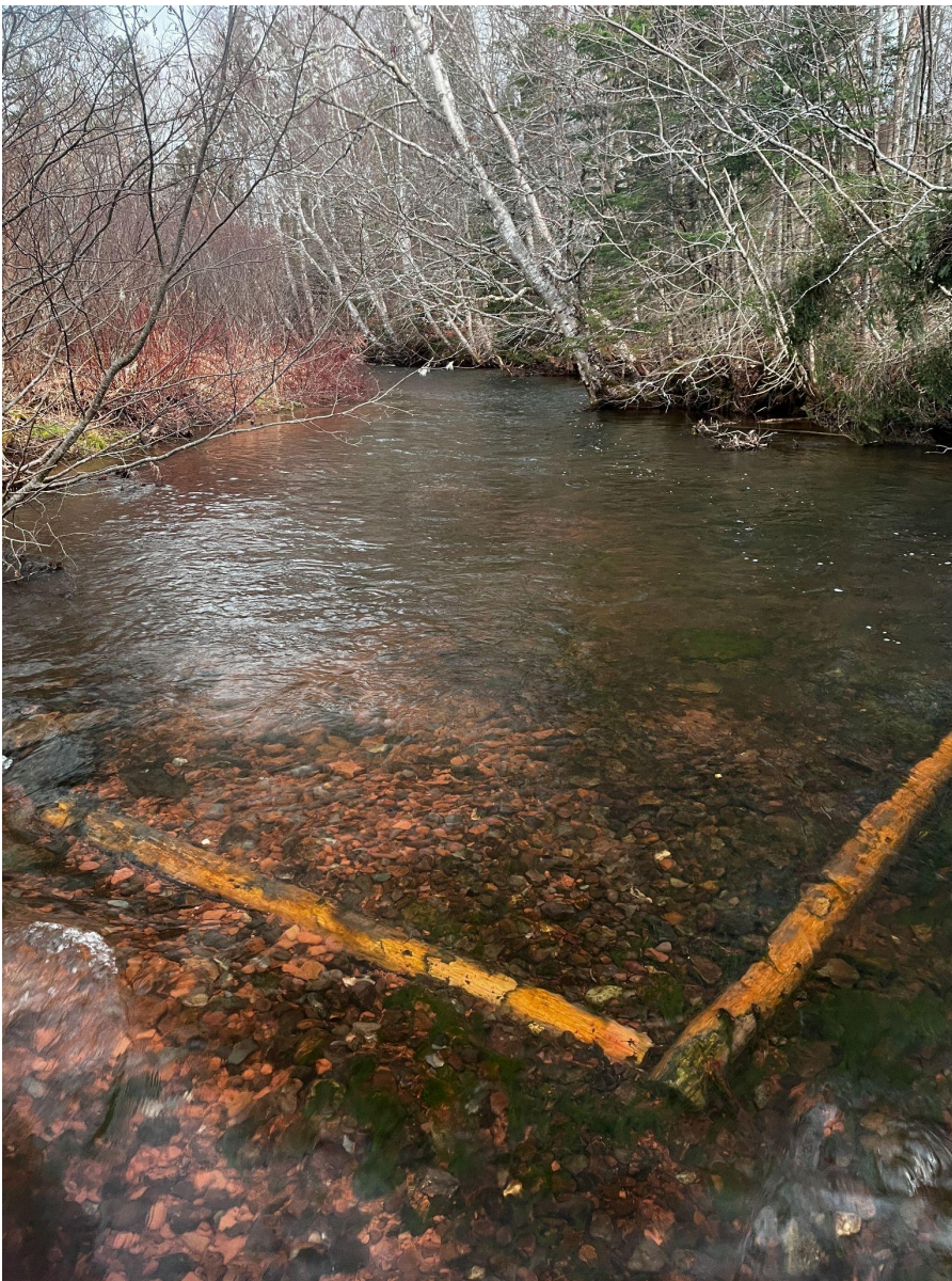
Photo on left displays an installed “V” spawning bed structure on the main West River with an Atlantic salmon redd. The photo on the right displays a “V” spawning bed structure on the upper main West River installed in 2023 and in 2024 it also had an Atlantic salmon redd utilizing it.
