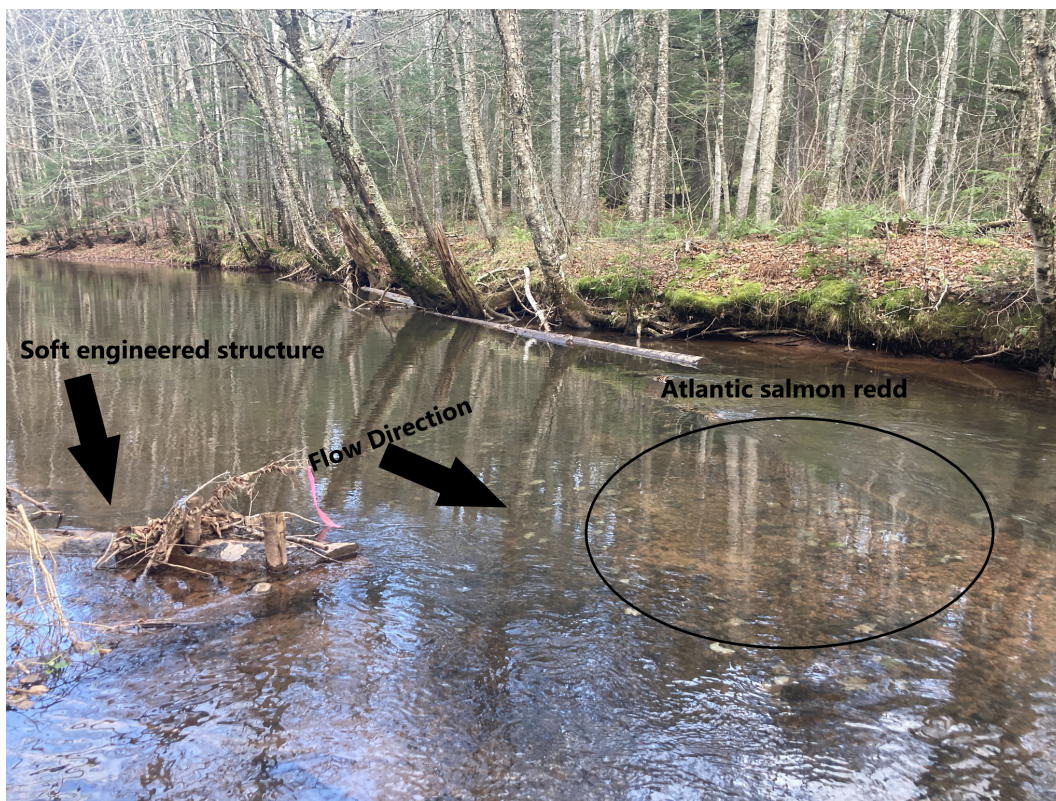
Image 1. This image shows a soft engineered structure installed by CQWF to help alter flow characteristics and encourage salmon to spawn over an area with high quality substrate.
