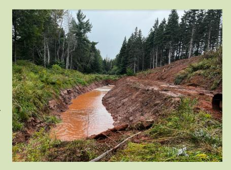
on the Clyde River a sediment trap was re-excavated on the west branch permanently removing 300 m<sup>3</sup> of sediment.
