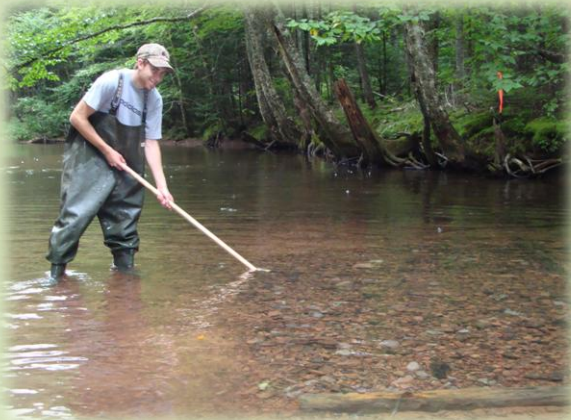
Summer student Kyle Doucette rakes new gravel / cobble mix in restored river bed
