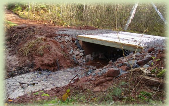
New ATV bridge built by CQWF in 2013 to replace a badly damaged culvert.
